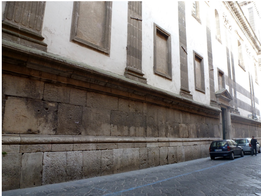
3. Capua, church of the Annunziata, Detail of the base constructed with the ancient blocks from the amphitheatre
